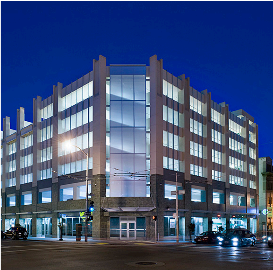
Images of UC Hastings parking garage located at 376 Larkin Street
